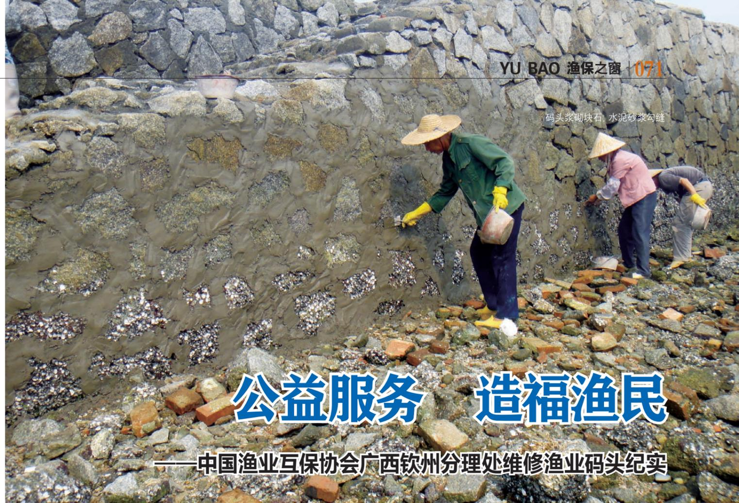
码头浆砌块石，水泥砂浆勾缝
